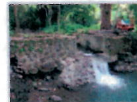
The fish passage structure was modified to provide a rock refuge that native species can ascend, while continuing to exclude non-native aquatic species. Photo: Gordon Smith, FWS
