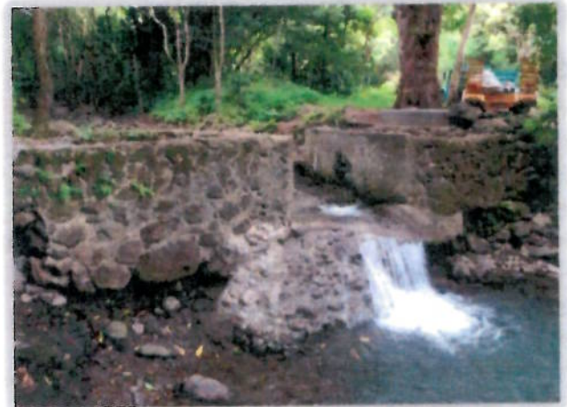
The instream structure was modified to provide a rock surface that native species can ascend, while continuing to exclude non-native aquatic species. Photo: Gordon Smith, FWS
