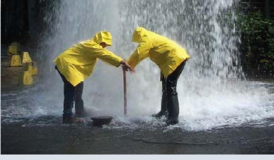
Finding: BWS pipelines suffer deterioration from age, corrosion, and soil, leading to more than 300 water main breaks per year.
