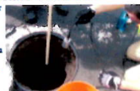
Echologics staff inserting a sensor onto a 42-inch water main.
